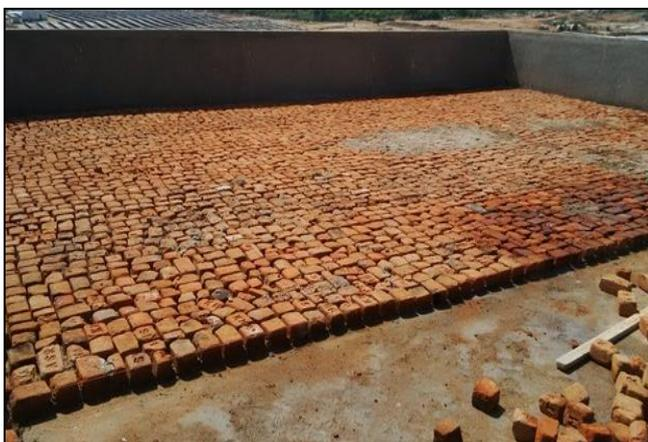
**Fig 3:** Laying of brick bats
