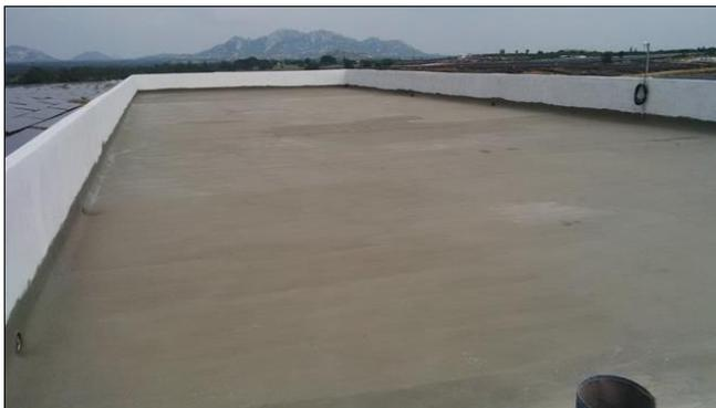
Fig 6: Final layer finishing surface of bricks bats water proofing
