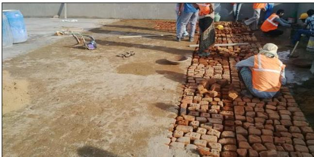
Fig 5: Bricks lying and mortar filling for each layer
